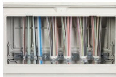
▲ Pedestal with open cover and micro-duct pipes fitted
