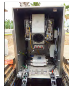
Underground distribution system EK 890 – open
