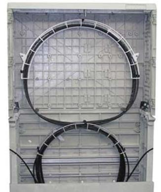
Fig.: Cabinet with fibre optic cable
